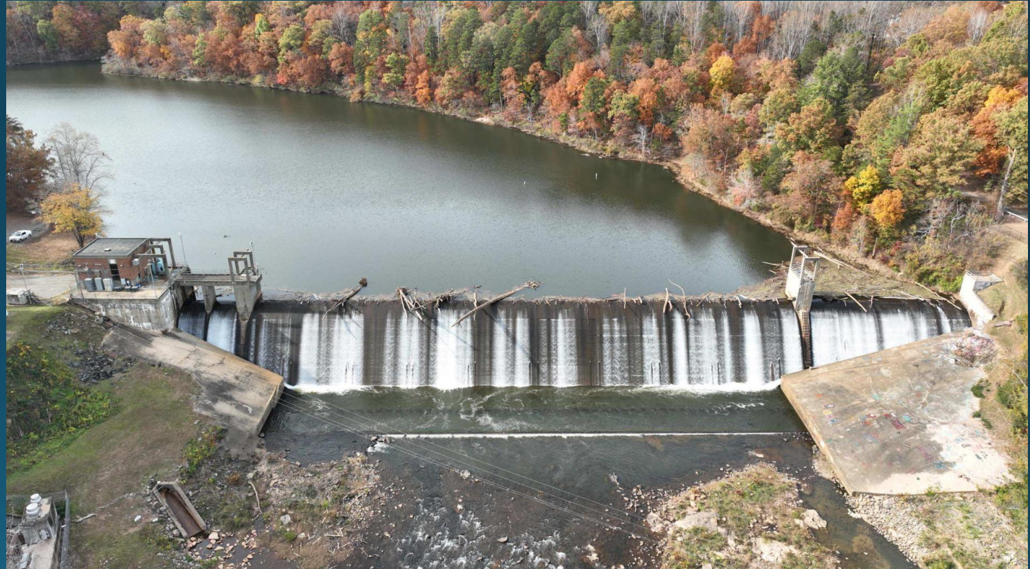
South Fork Rivanna Reservoir Dam
