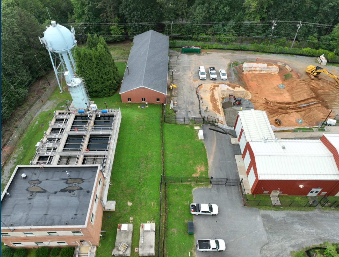
Excavation for new GAC Building and Clearwell
