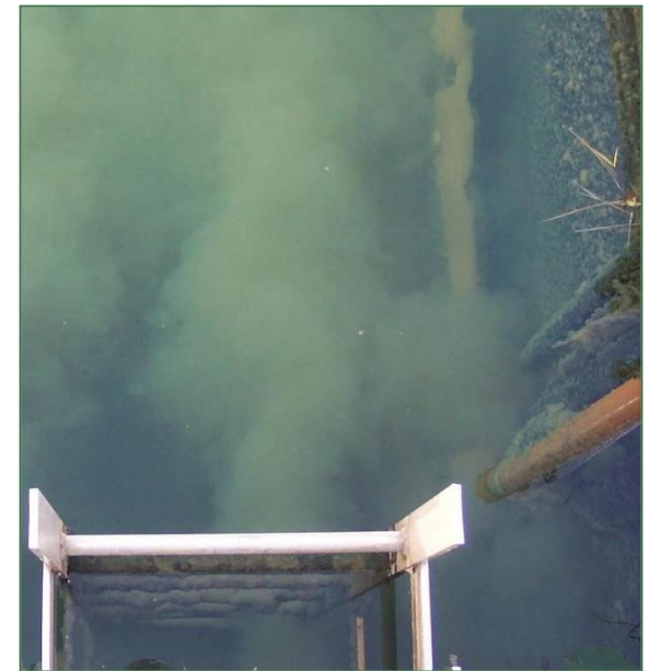
Flocculated particles entering sedimentation basins
